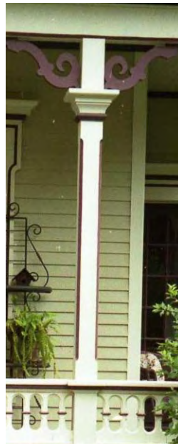
Italianate Porch post with stop chamfers
