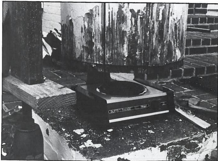
Three four-foot 2 × 10s bolted to each column (left), provided a triangular lifting jig for the hydraulic jacks. Electric heaters dried out the column interiors while the bases were patched and consolidated.
