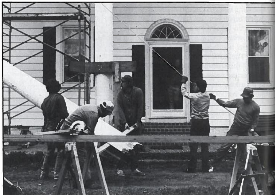
Removing the "worst case": Plunge-cutting the shaft makes room for a 2×4 handle. Then, by rigging with a block-and-tackle, the entire column is lowered to the ground.
